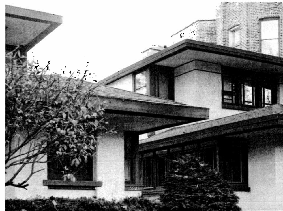
THE PRAIRIE-STYLE ARCHITECTURE OF THE GAULER TWIN HOUSES IS IN MARKED CONTRAST TO NEIGHBORING THREE-FLATS OF THE SAME PERIOD. THEIR DISTINCTIVE FEATURES INCLUDE DEEP OVERHANGING EAVES, RIBBONS OF WINDOWS, AND ROUGH-TEXTURED STUCCO WALLS.
